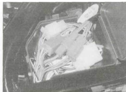
19.3c On FZS models, the wiring connectors are in the black box
